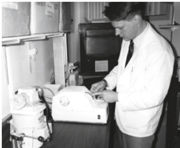
FIGURE 15-3 Hand-polishing of lens edges.
